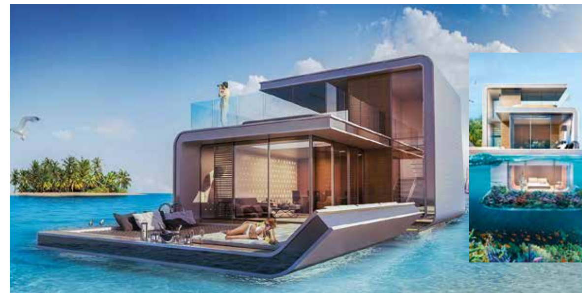
The Floating Seahorse villas (42 villas), Dubai, U.A.E.
